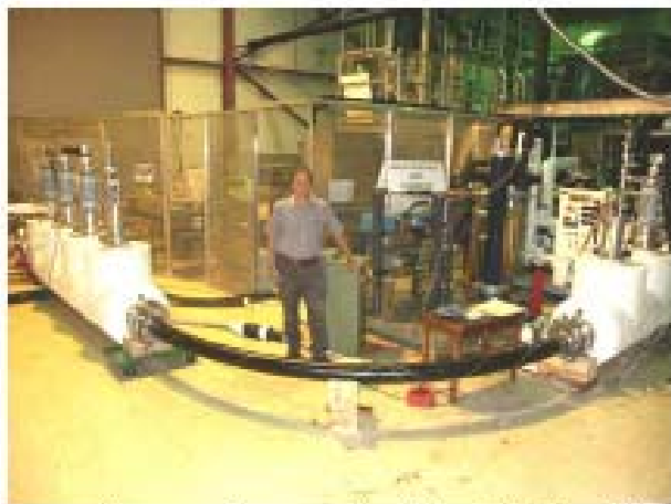
Testing 90 degree tri-axial cable bend in HTS cable test facility at ORNL (2005)
